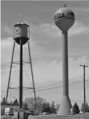
1985 Through the CDBG program, the first elevated water storage tank was built in the City of Vega in Oldham County. Fifteen years later, the City replaced the tank.
