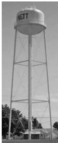
1990 The City of Stinnett received its new water tower.
